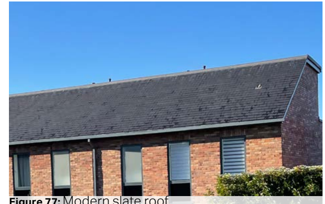
Figure 77: Modern slate roof
