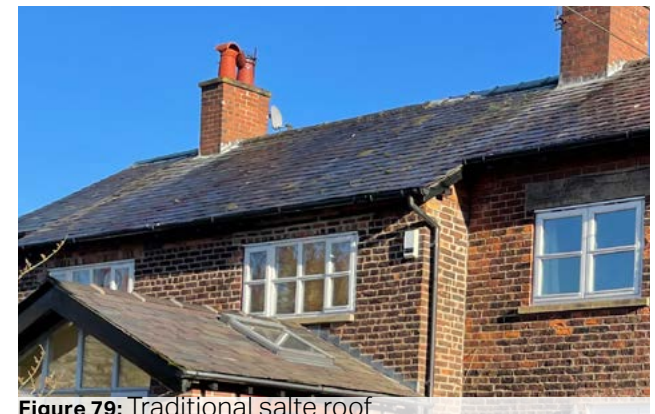
Figure 79: Traditional salte roof
