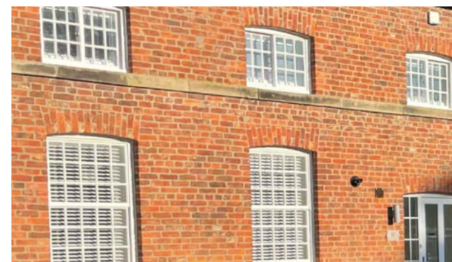
Figure 91: Arched brick lintel with a stone sill string. Windows have timber glazing bars
