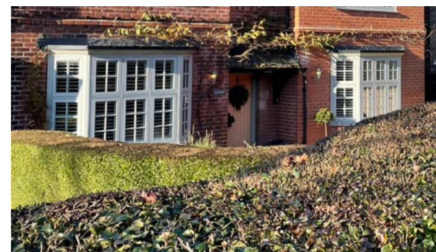
Figure 101: Timber bay windows with glazing bars
