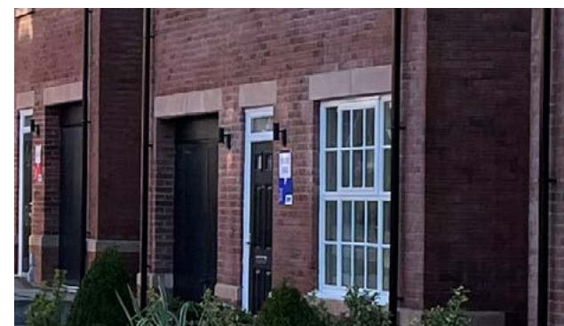
Figure 102: Casement windows with glazing bars and stone sill and lintel
