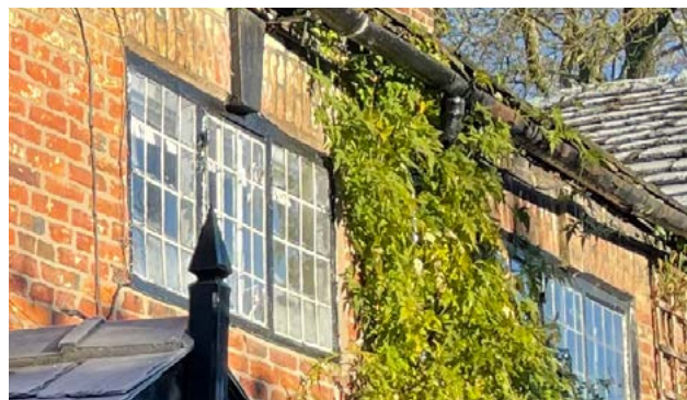
Figure 88: Traditional timber framed windows with lead glazing bars
