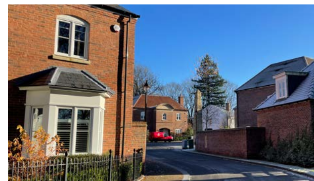
Figure 93: Bay window with a slate roof
