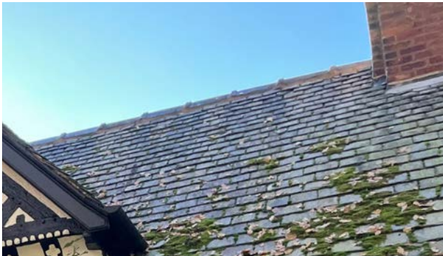
Figure 86: Natural slate roof with diminishing slate sizes
