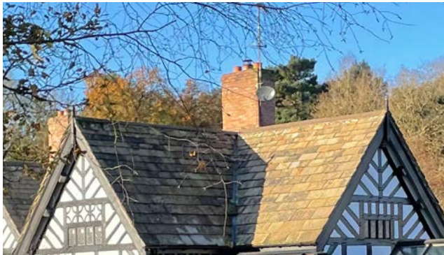
Figure 87: Traditional stone roof
