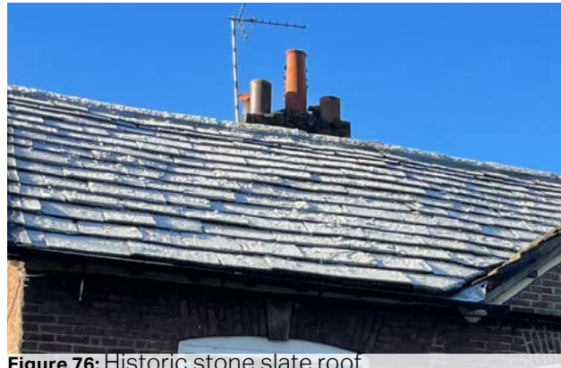
Figure 76: Historic stone slate roof
