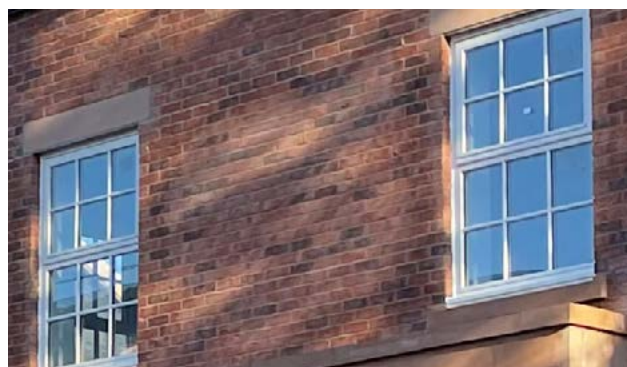
Figure 92: Mock sash casement windows with glazing bars and stone sill and lintel
