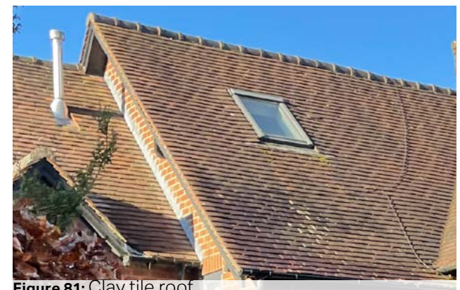
Figure 81: Clay tile roof
