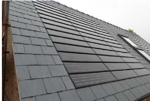
Figure 132: Contemporary solar panel design can be subtle by integrating with a traditional roofscape.
