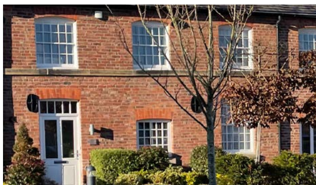
Figure 99: Arched windows with glazing bars and a stone window sill string shared along upper windows
