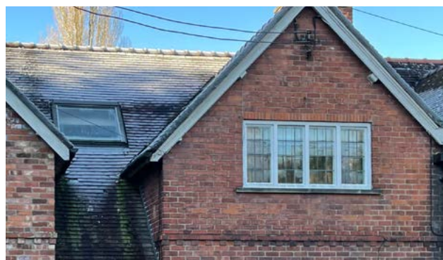
Figure 90: Timber casement windows with lead glazing bars and a stone sill
