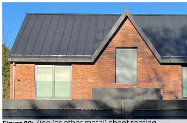
Figure 80: Zinc (or other metal) sheet roofing
