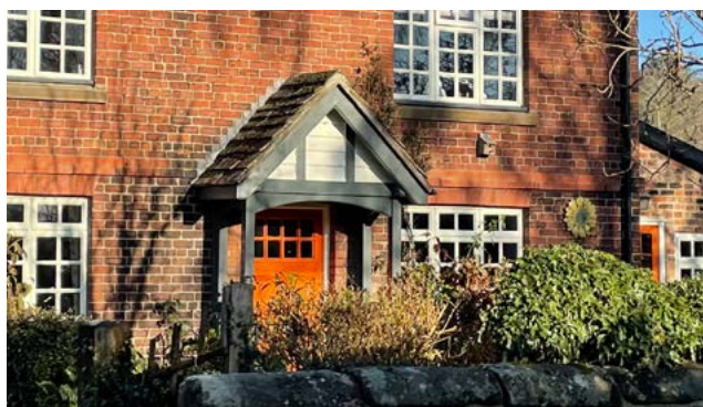
Figure 96: Timber framed covered porch with tiled roof
