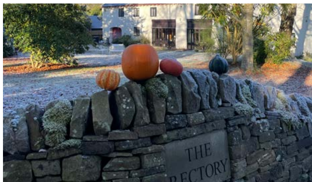
Figure 103: Drystone wall boundary
