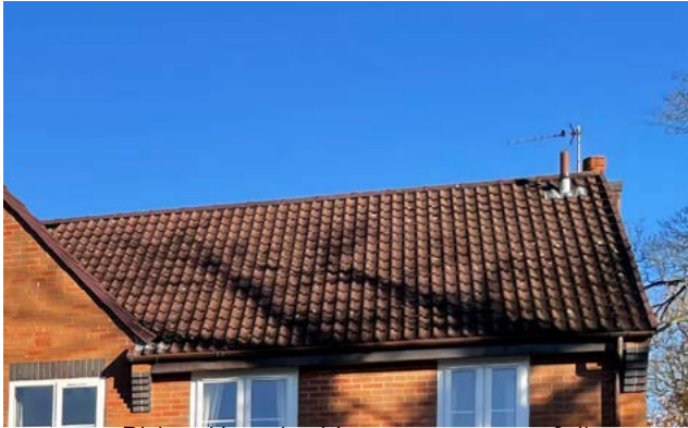
Figure 84: Ridged interlocking concrete roof tiles
