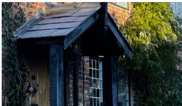
Figure 95: Timber framed covered porch with a slate roof
